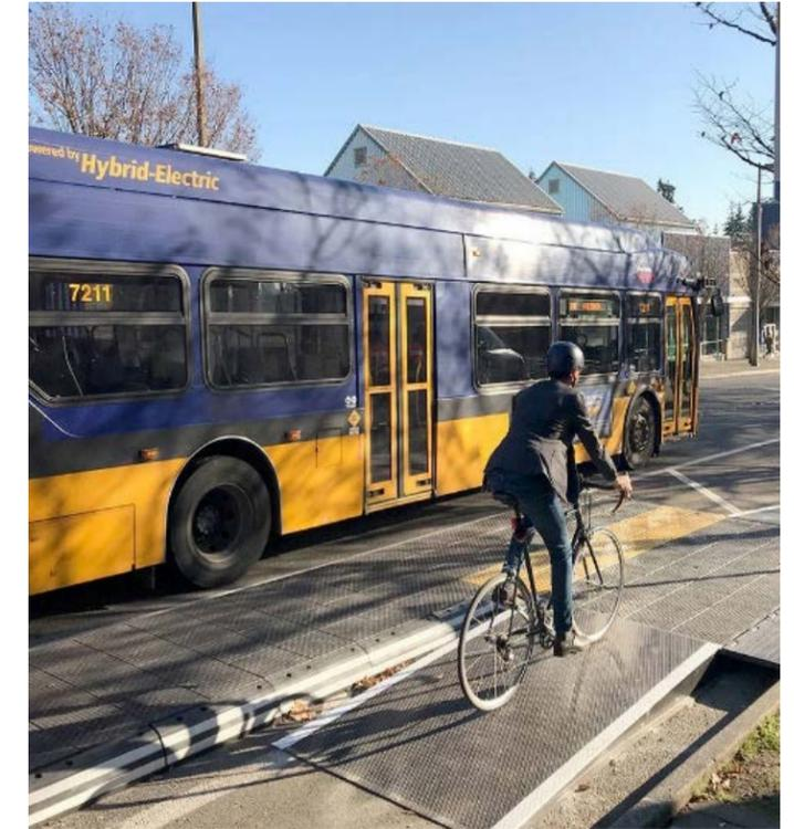
The new bus platform is installed on 108th Avenue NE, south of NE Second Street. It is made of 300 interlocking plastic panels that snap together, allowing for its rapid installation.
