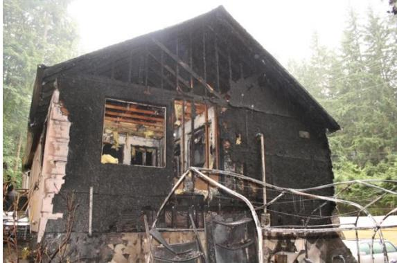
7/31/2011 – This single family home is also the site of a biodiesel manufacturing facility. This fire resulted in an estimated loss of \$400,000 and originated in the vicinity of the biodiesel reactor.
