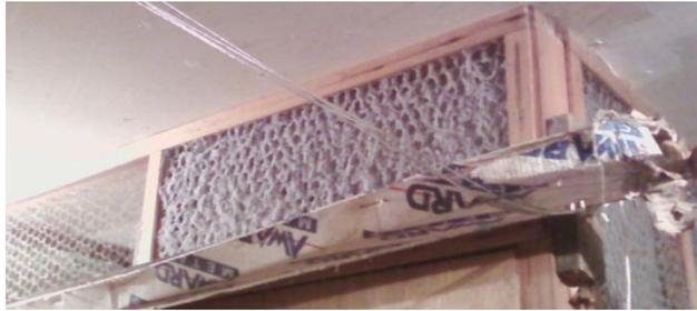
A disconnected dryer vent led to lint accumulations in a storage room of a multi-family building. In the same building, smoke detectors were missing in the bedrooms and a number of smoke detectors in other locations lacked batteries.
