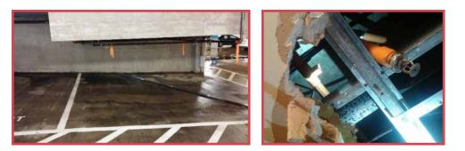
sheared off as a result (See photo). The dry sprinkler system activated, which also caused the primary fire pump to engage. Simultaneously,
