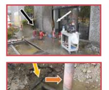
Two workers were in the process of brazing a copper water line in a ditch when a fire erupted. Both workers suffered significant burn injuries and were transported to area hospitals.
