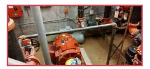
The primary and secondary fire pumps and controllers resulted in failure when the fire pump room filled with water and damaged the electric motors and components (see photo). The water reservoir automatic fill sensor reportedly detected low water in the tank, which subsequently overfilled the reservoir and pump room. Standing water
