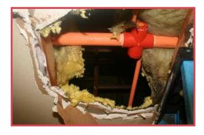
A fracture to the ¾" branch line on the CPVC sprinkler pipe occurred at the multifamily dwelling when maintenance personnel were working in the attic and reportedly stepped on the piping that was tented with insulation (see photo). Water flowed from the sprinkler piping until responding units could locate and turn off the control valve. Twelve living units were evacuated and deemed non-livable until building repairs were made due to water damage.
