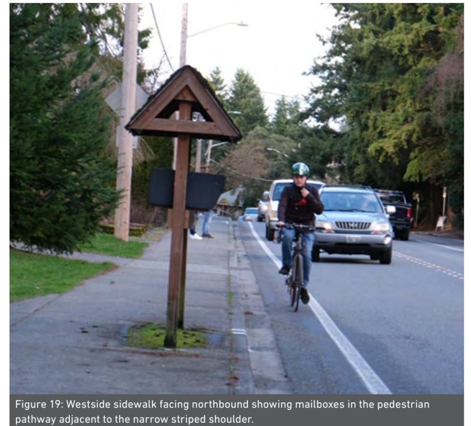
Figure 19: Westside sidewalk facing northbound showing mailboxes in the pedestrian pathway adjacent to the narrow striped shoulder.
