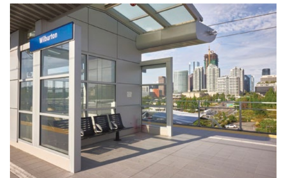
The 2 Line passing through Wilburton is among the advantages of the neighborhood for sustainable practices.
