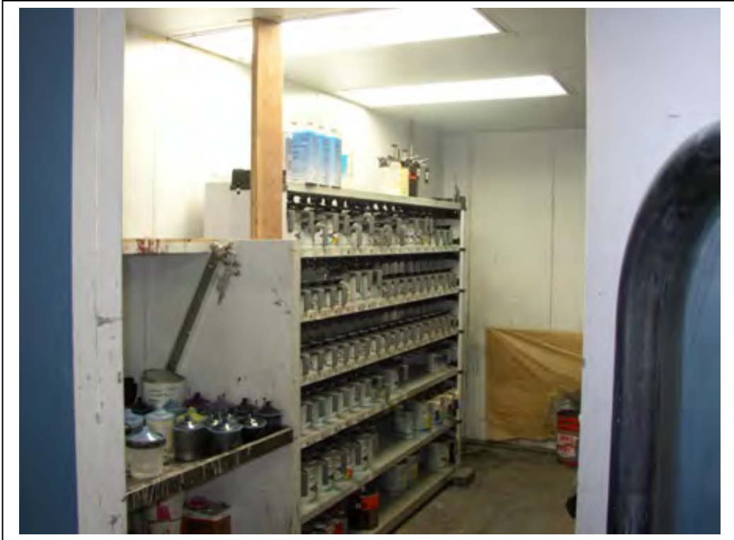
Photo 8: Paint storage room inside subject building.
