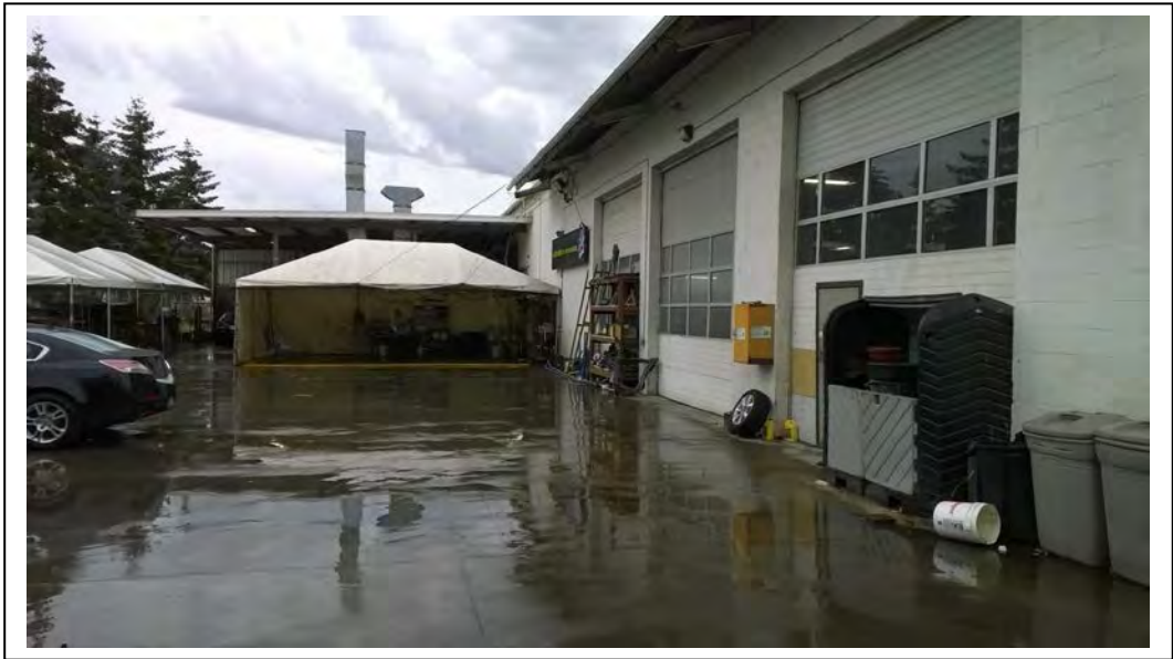
Photo 5: View looking south along east side of subject building towards detailing pad.
