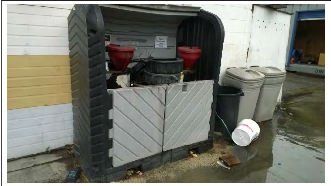
Photo 6: Used oil containment device along east side of subject building.
