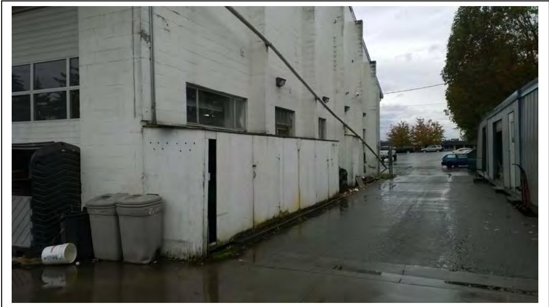
Photo 4: View of north exterior of subject building (looking west).
