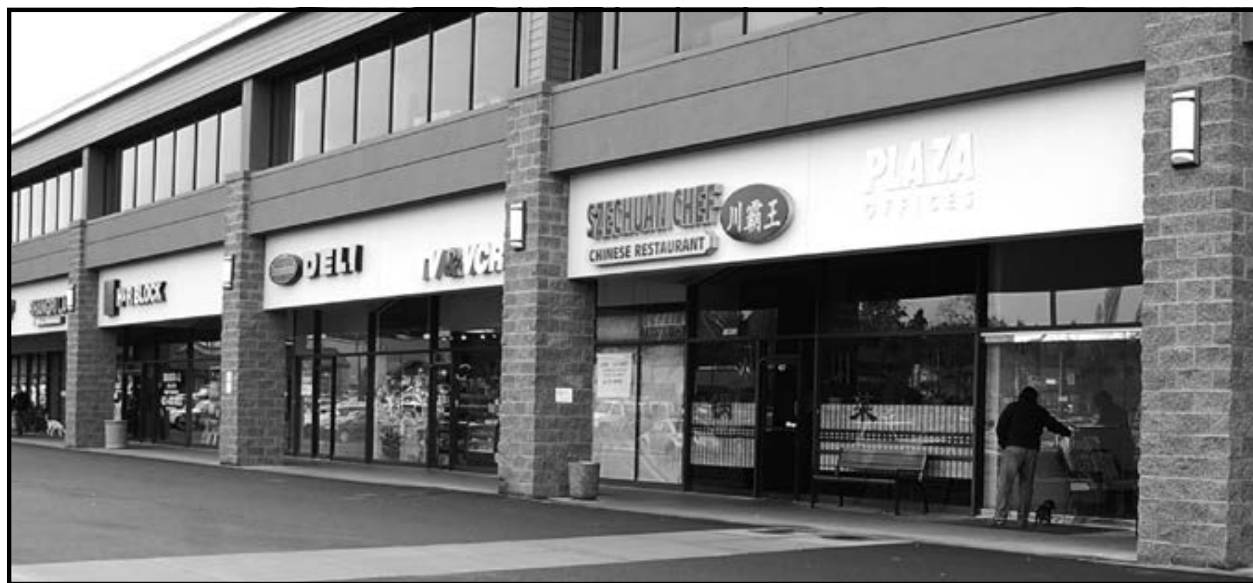
The revival of Kelsey Creek Center, a highlight for East Bellevue, was a part of the city's vision for the area.
