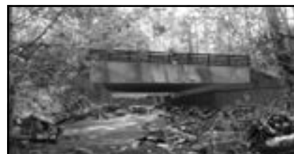
New Coal Creek bridge Page 5
