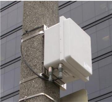
*Bluetooth travel time collection hardware will be installed at four locations on Main Street.*
