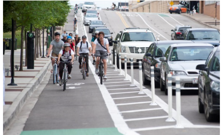
Parking, Painted Buffer, and Post Separation
