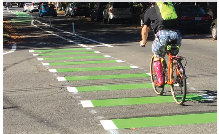
Green Pavement Markings
