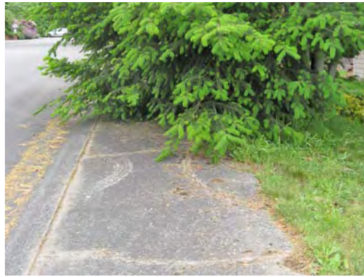
SE 20th Street & 140th Avenue SE.
