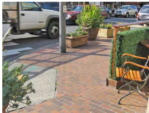
Furniture and planters at sidewalk café obstruct ramp landing and narrow the pedestrian pathway at 102nd Avenue SE & Main Street.
