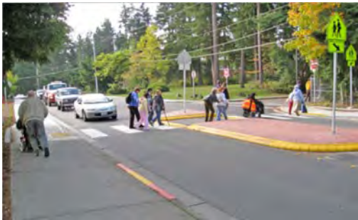
Pedestrian median with a cut-through design provides people with disabilities a point of refuge when crossing at 164th Avenue NE south of NE 24th Street.
