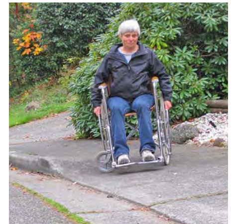
Steep driveway cross slope.
