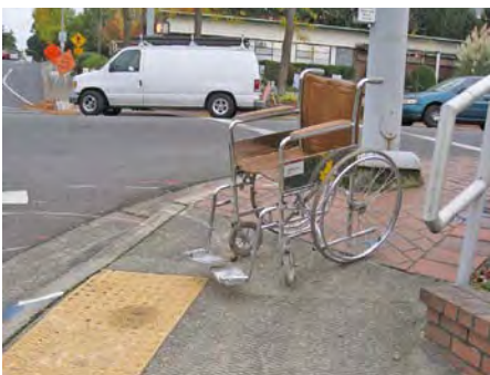
Steep ramp flare slope.
