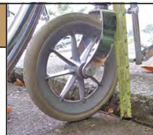
Change in sidewalk level (2 inch) at 148th Avenue NE & NE 35th Street.
