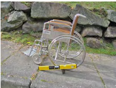
Sidewalk grade of 22% on 166th Avenue SE between Phillips Road and SE 39th Place.
