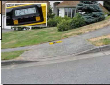
Steep ramp landing panel slope at SE 56th Street & 175th Place SE.
