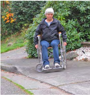
A series of driveway apron flares with 11% cross slope measurements at 130th Avenue SE & SE 26th Street.
