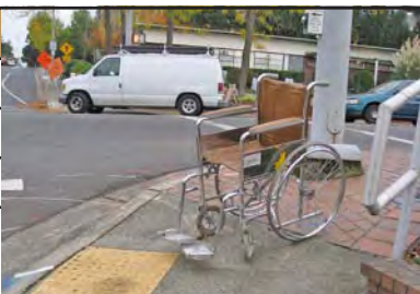
Steep ramp flare slope at Main Street & 100th Ave SE.
