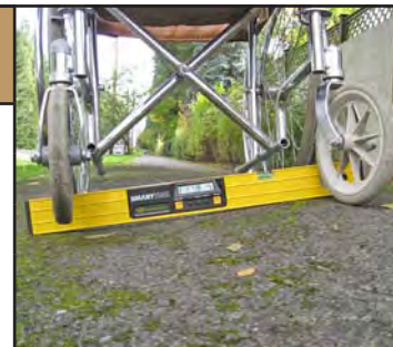
Example of 18 percent cross slope at NE 24th Street & 167th Avenue NE.
