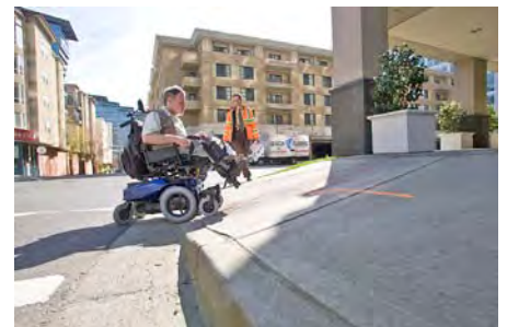
Steep ramp running slope.
