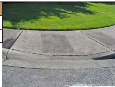
Non-standard detectable warning surface at SE 34th Street & 111th Avenue SE.
